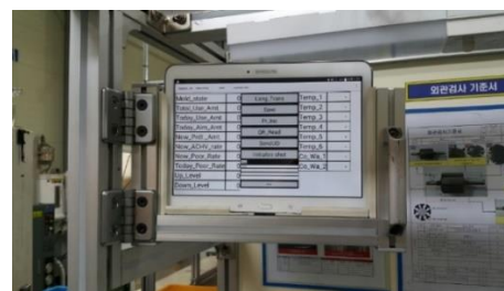
(b) Installed Teblet PC
