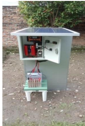
Figure 3. Battery charging process using a solar panel system
