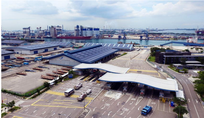
Figure 5. PVs covered on the warehouse roof space [53]
