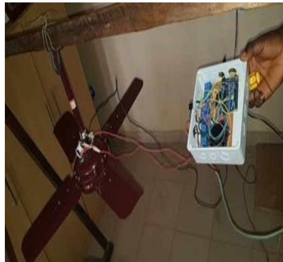
Figure 9. Image of the completed work
