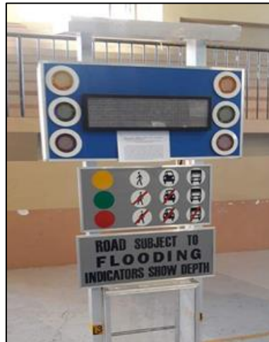
Figure 4. The road flood warning system
