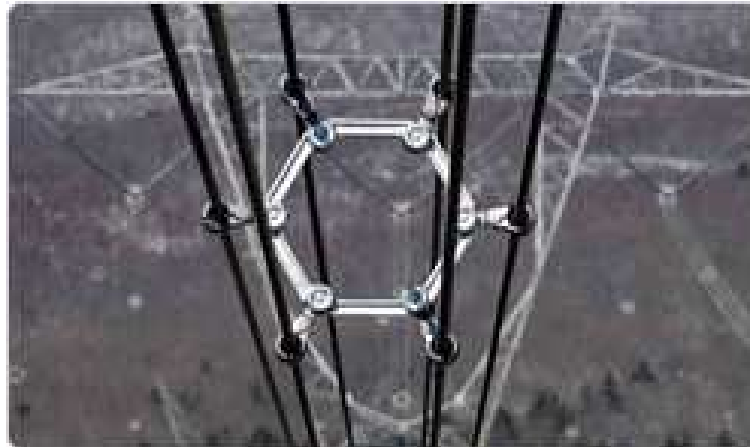
Figure 1. Six-wire transmission line
